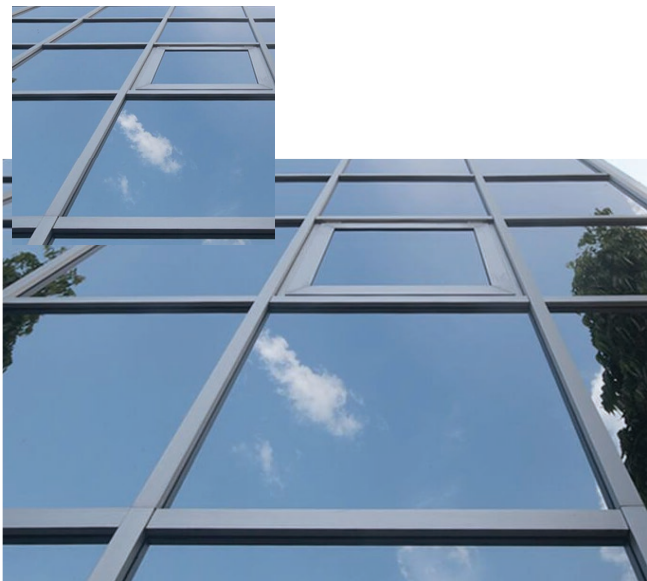
Visible frame or Standard: On the outside, the glazing is divided by horizontal and vertical lines formed by aluminum profiles of 50mm width.
